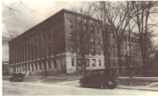
The continuing expansion of the Engineering Department called for the addition of another engineering classroom building across the street from West Engineering Building. The East Engineering Building, erected in 1922 provided classroom and lab space.
