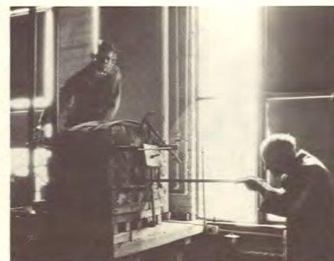
In the 1920s and '30s researchers investigated the uses of manufactured gas. Three specific projects were issues of heat treatment, decarburization of steel, and core baking.
