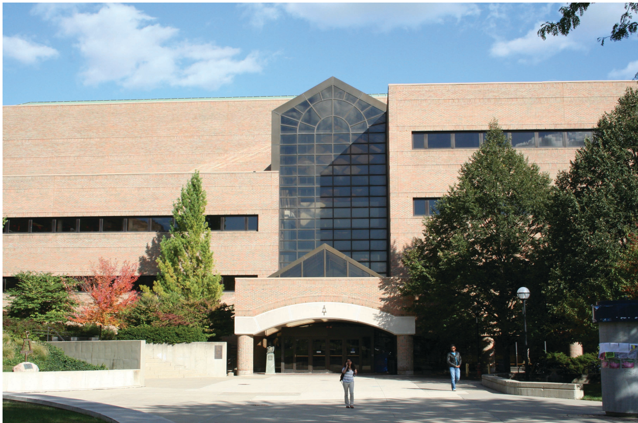
Fig. 2: West side of EECS Building
