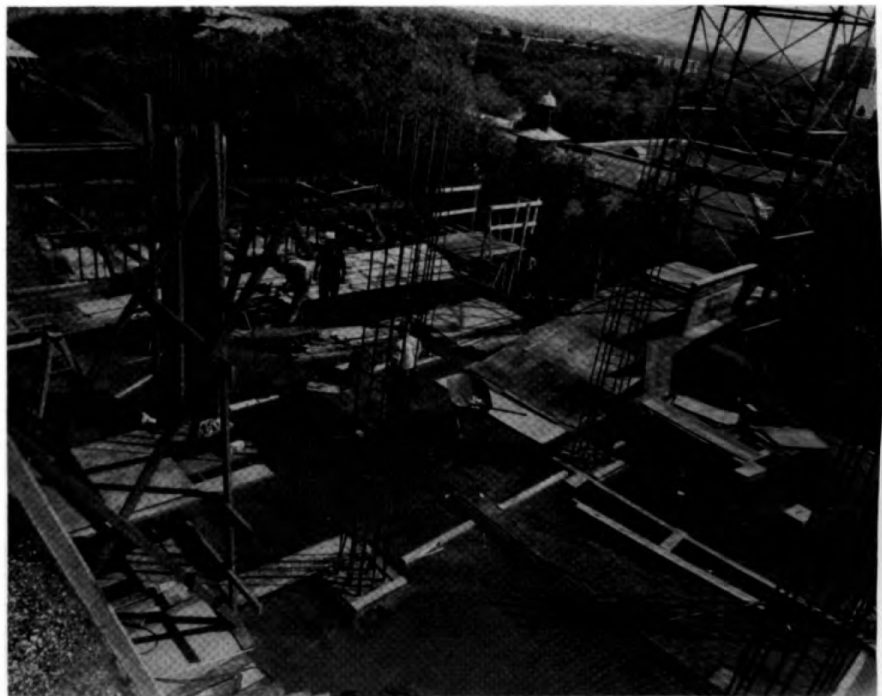
Construction on the General Library Addition.
